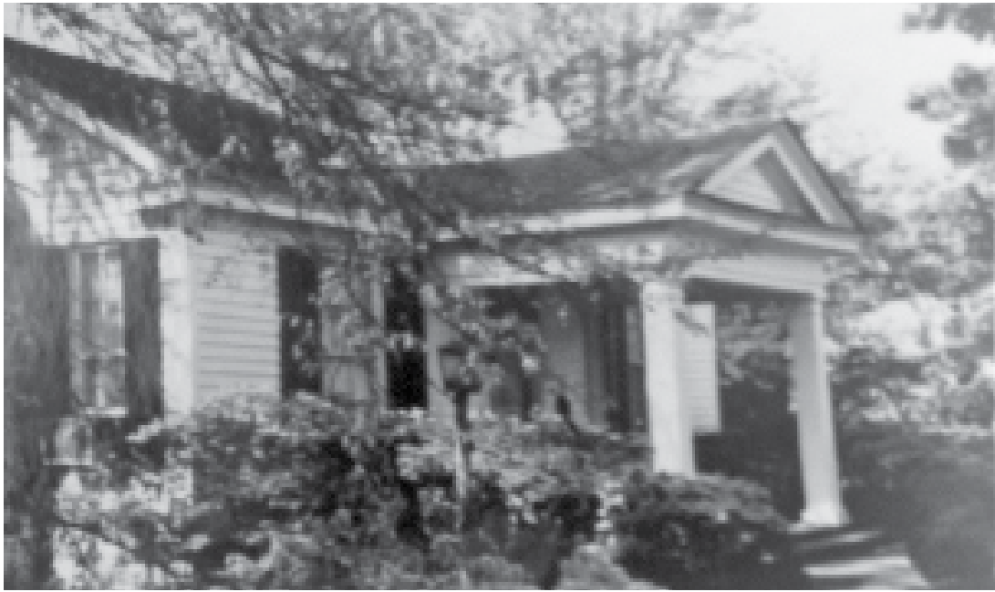
The McCarroll house, where the McCarroll/Francisco family has lived continuously for more than 155 years.
