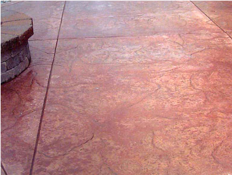
On this job, the orange release almost entirely covers the base color.
