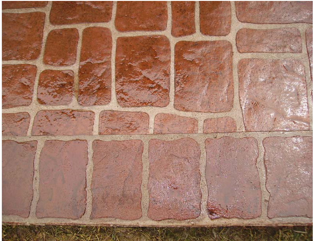
Real blocks don't have a mortar joint on the outside. Plan the job so it looks realistic.
