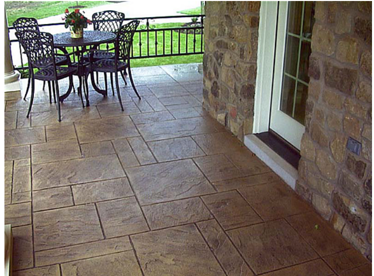
A proper amount of release was left on this job, so the dark walnut color remains only in the joints and depressions and the high spots show only the base color.
