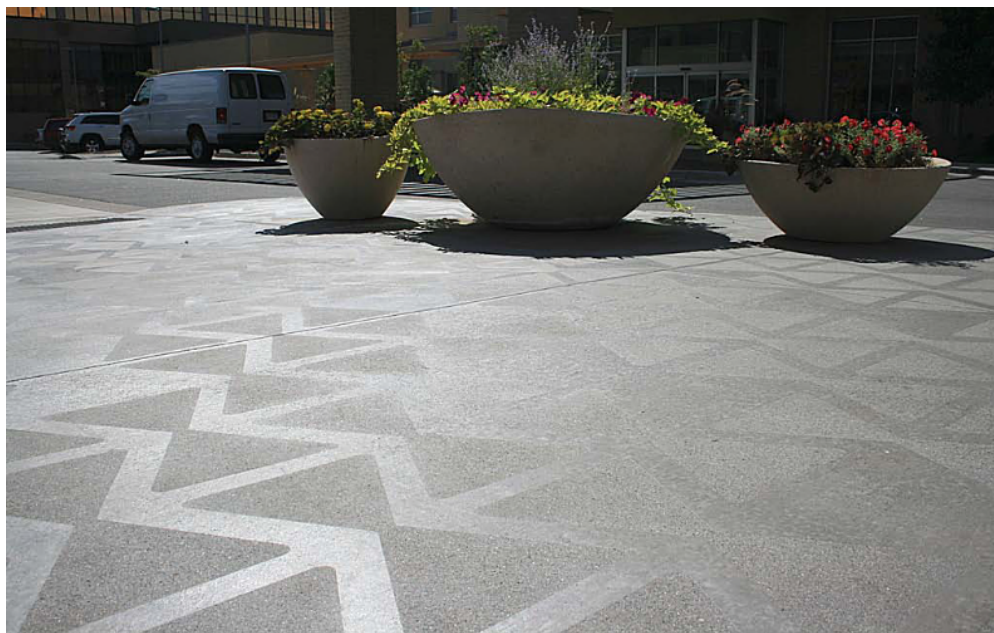
Subtle shifts in color and texture appeal to designers and owners in Colorado. Template sandblasting is one of the methods used to achieve this look.
