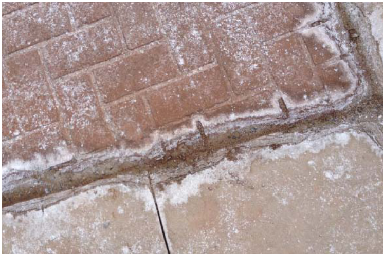
Water from freeze-thaw cycles and damage from de-icers have weakened a joint and deteriorated the concrete.
