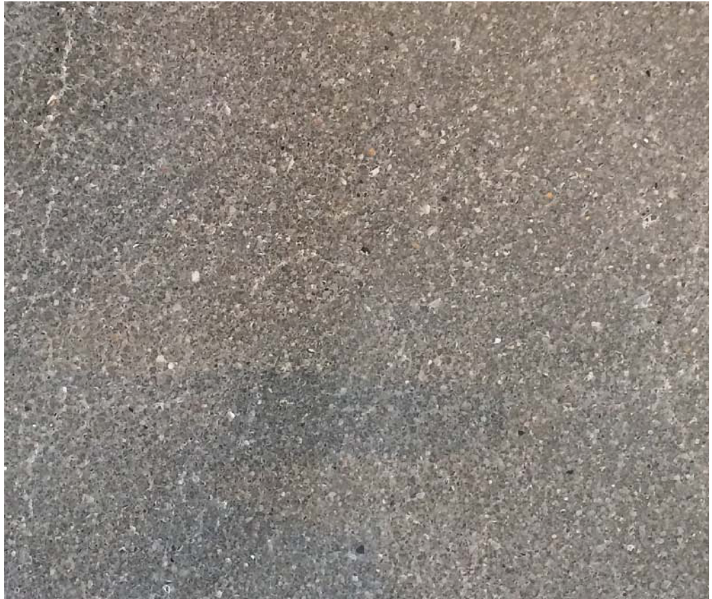
Seen here is a salt-and-pepper reveal with no small aggregate. There must be small to medium aggregate exposure or it is a CCAA Aggregate Exposure Class B- Fine/Sand Aggregate Finish.
