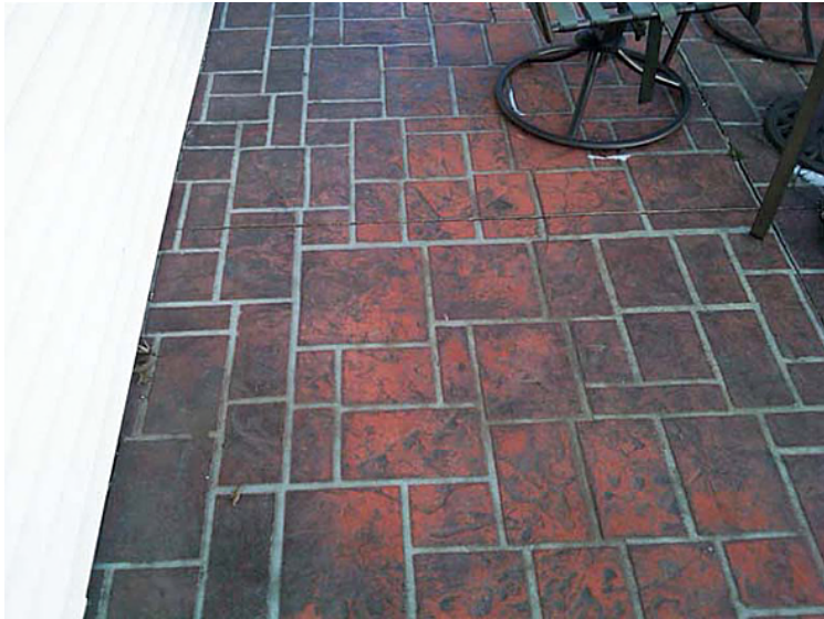
Excess charcoal release lifted off when the sealer failed, leaving a blotchy surface.
