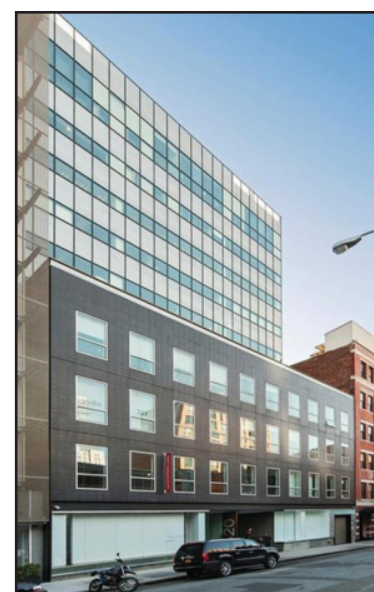
520 West 27 th Street (between 10 th and 11 th Sts.) - Manhattan, NY
