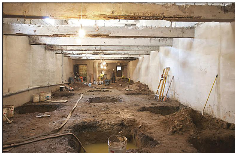
Basement, before redevelopment.
