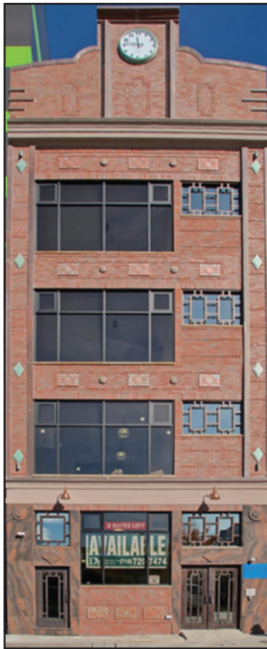
After: 22-07 41 st Avenue - Long Island City, NY
