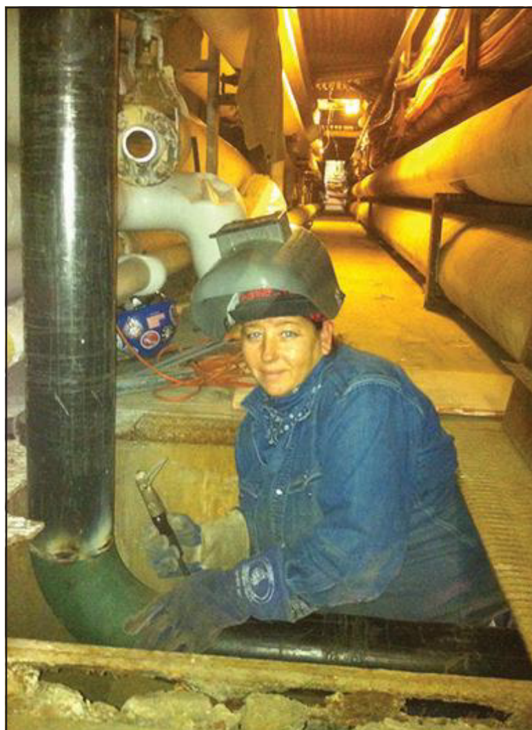
Powers welding main steam piping at Rockefeller University.
