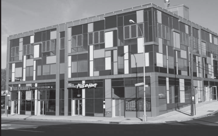
Intricate curtain wall - multiple panel types, sizes and tints
