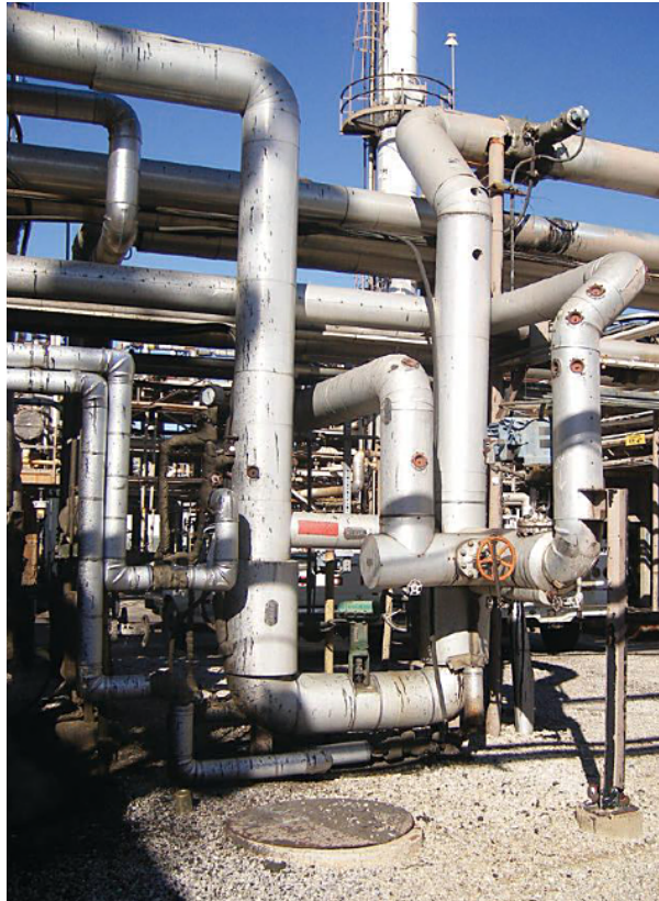
Above: Typical situation of an inaccessible manhole inside the refinery.
