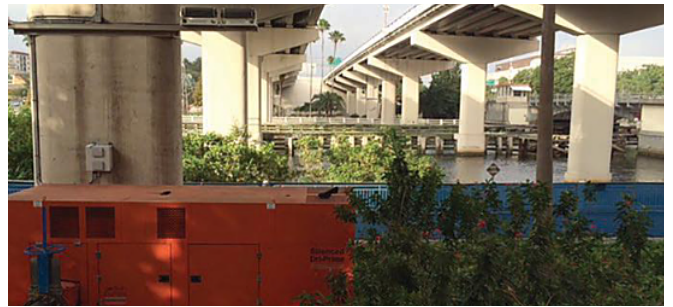
Top: The fuel cubes, lower right and left, were used as part of the back-up redundancy of the system for the diesel driven pumps. Bottom: Space was limited under the expressway and along the river.
