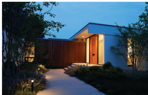
Renovated by Deborah Berke Partners in 2015, Milton Klein designed this 1960s house in Rye, NY
