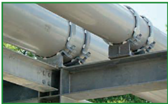
E-Z Line®'s In-house structural engineer and designers created supports based on axial, lateral, and vertical loads provided by our customers.
