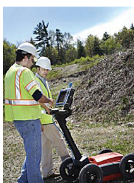
GPR units surveying the location of buried tanks at a gas station and looking for other underground obstructions.
