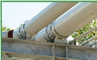
E-Z Line® Custom Pipe Shoes with I-Clip Liner and E-Z Line® Standard Pipe Shoes 2\" PS. with FRP Liner.
