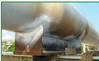
Custom Weld-on Pipe Shoes with Guides and Anchor Stops.
