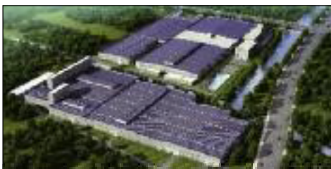
Novalis, with the first Chinese factory to export LVF into the global marketplace, is expanding its manufacturing facility outside Shanghai.
